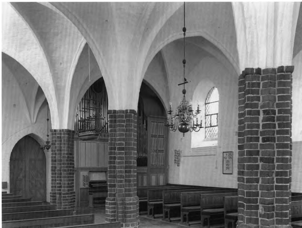
Fig. 47. Indre, set mod nordvest. NE fot. 1994. - Interior to the north-west.
