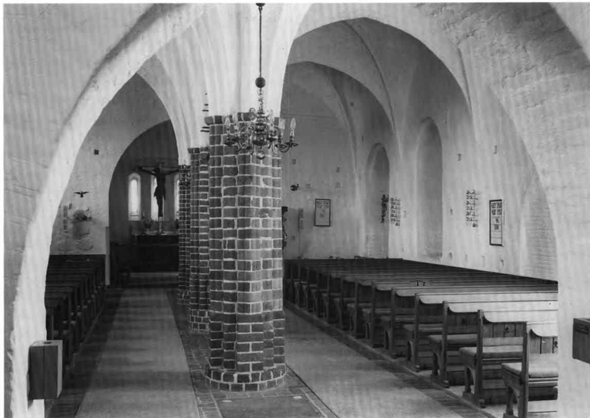
Fig. 16. Indre, set mod øst. LL fot. 1981. - Interior to the east.
